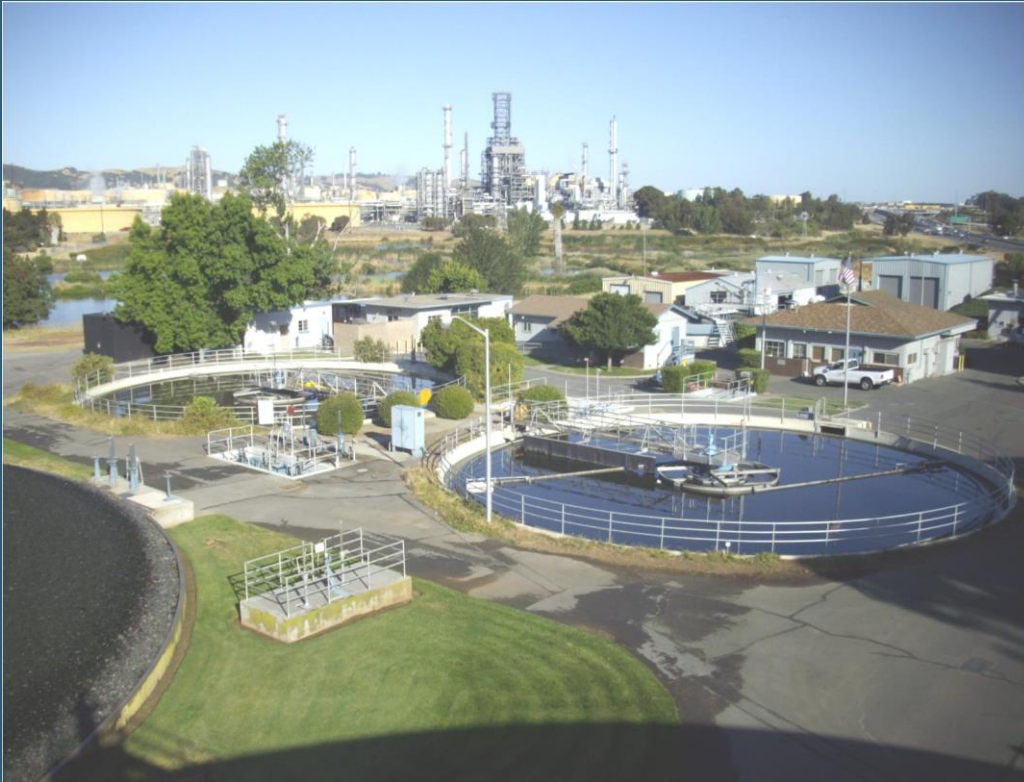
Wastewater Treatment Plant
