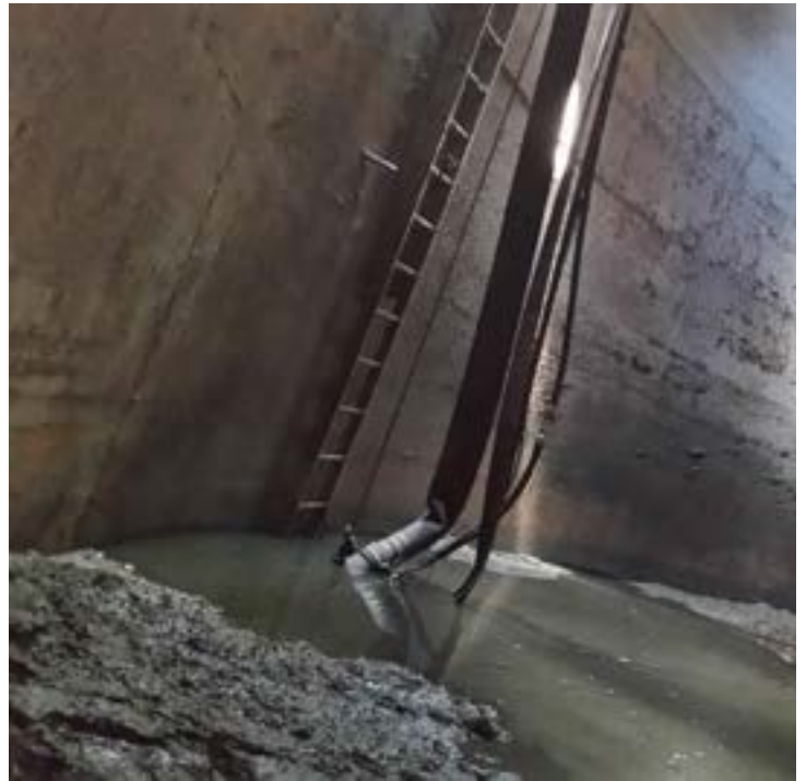
A view inside the empty Anaerobic Digester
