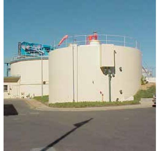
These digesters break down solids from the wastewater. It is an important part of the wastewater treatment process.
